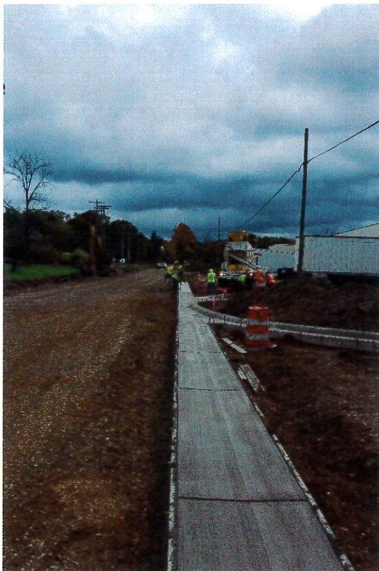
Placing Curb & Gutter Prior to Paving
