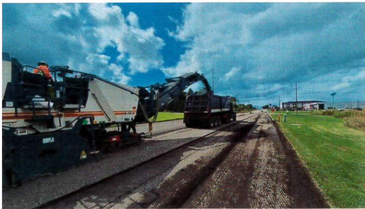
Milling Machine Removing Top Layer of Asphalt
