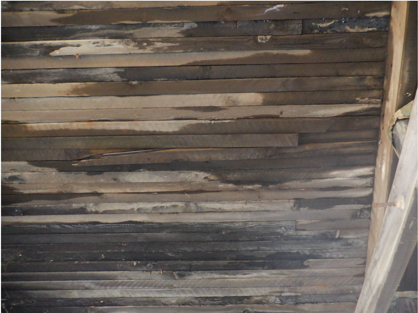
BROKEN DECK BOARDS IN CENTER SPAN NEAR EAST PIER
