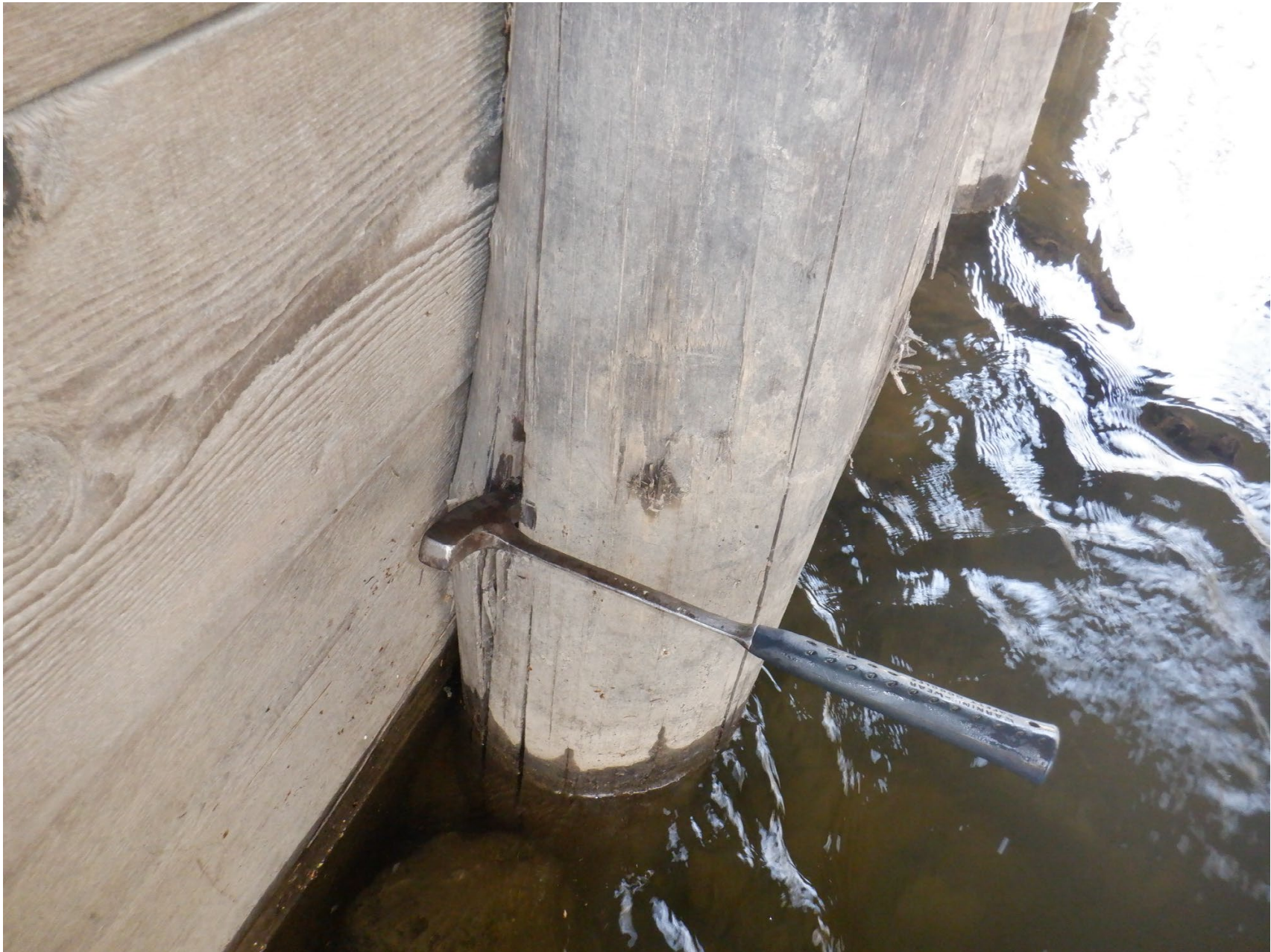
EAST ABUTMENT PILE 4N ROTTING ON BACKSIDE NEAR WATERLINE
