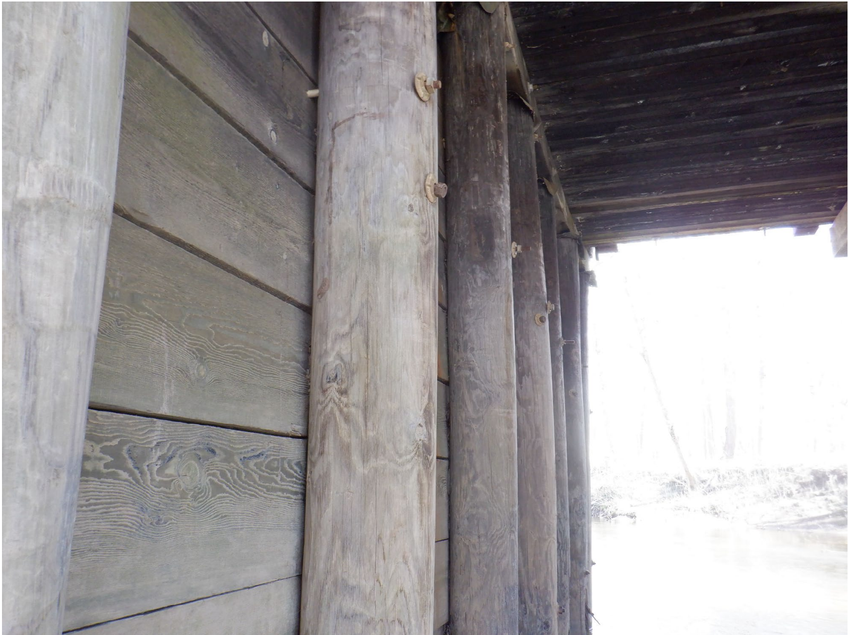
WEST ABUTMENT PILES BOWED IN NORTH HALF
