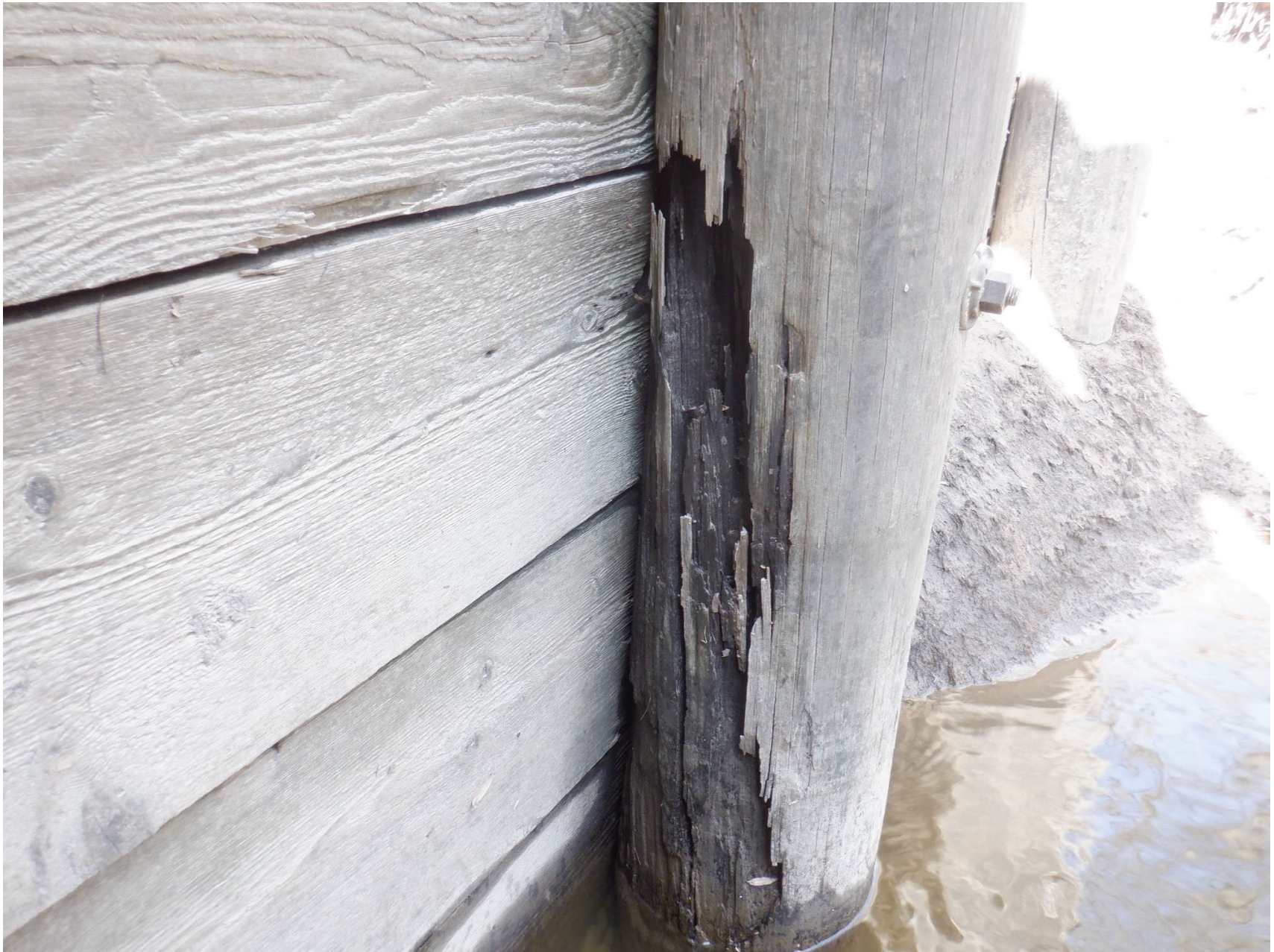
NORTHWEST WINGWALL PILE ROTTING
