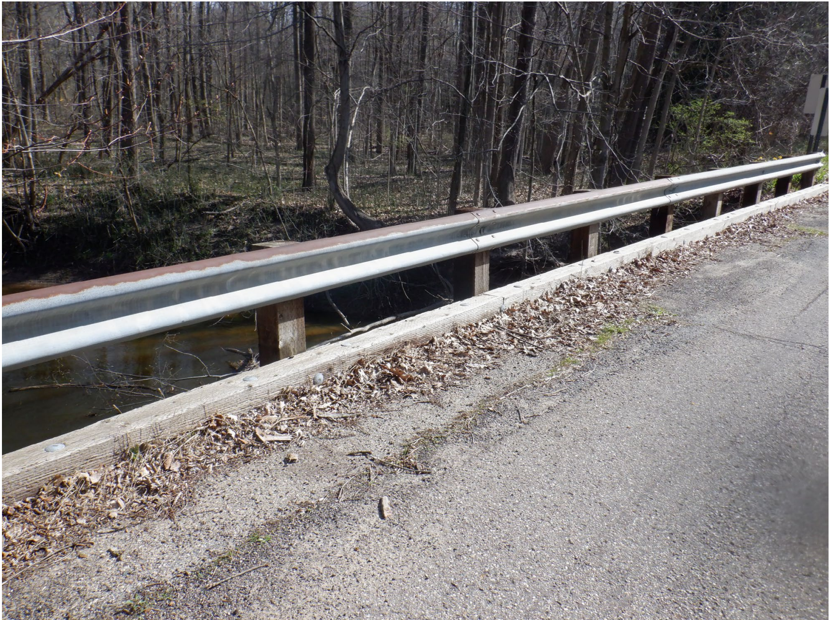
NORTH BRIDGE RAIL, W-BEAM RUSTING, NEWER POSTS AND BRUSH BLOCK
