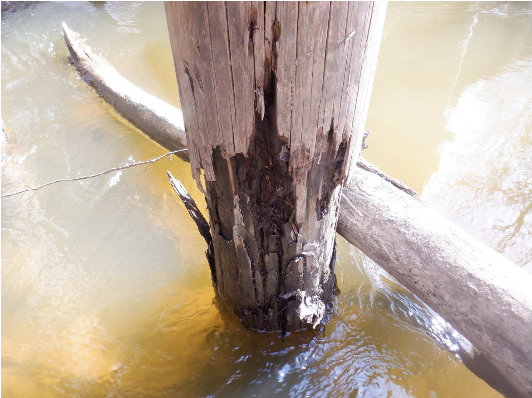
OUTER 1"-2" ROTTING ON WEST PIER PILE 1S
