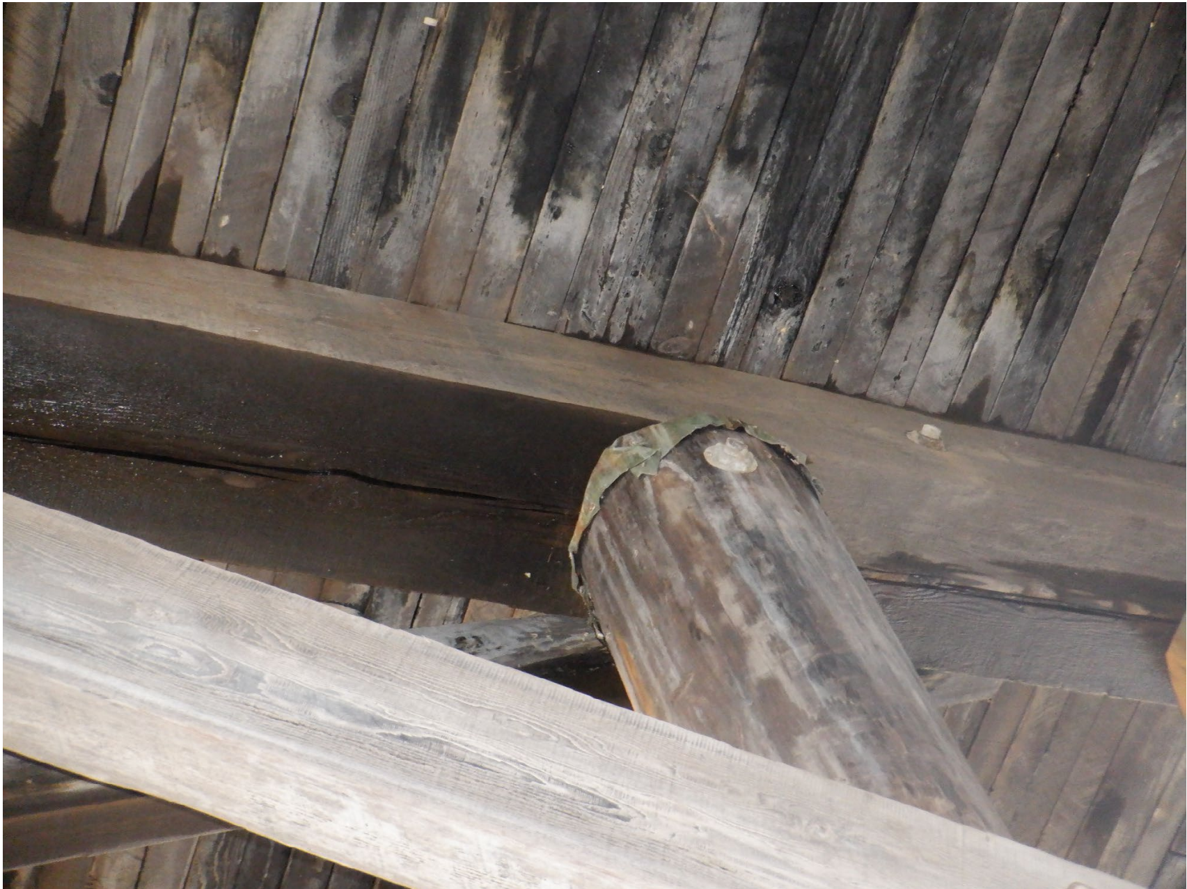
SPLIT WITH LEAKAGE ALONG BOTTOM OF EAST PIER CAP
