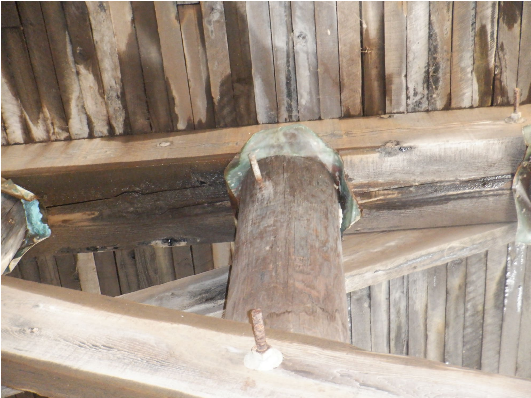
CHECKING WITH LEAKAGE ALONG BOTTOM OF WEST PIER CAP
