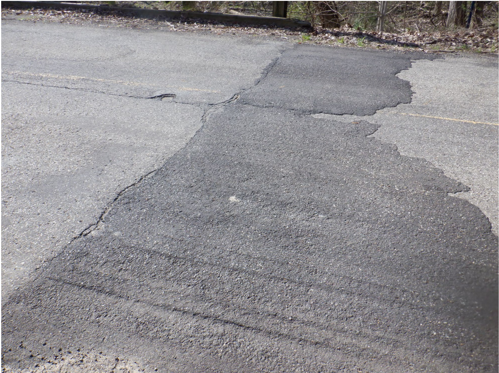
NEWER HMA WEDGING ON WEST APPROACH
