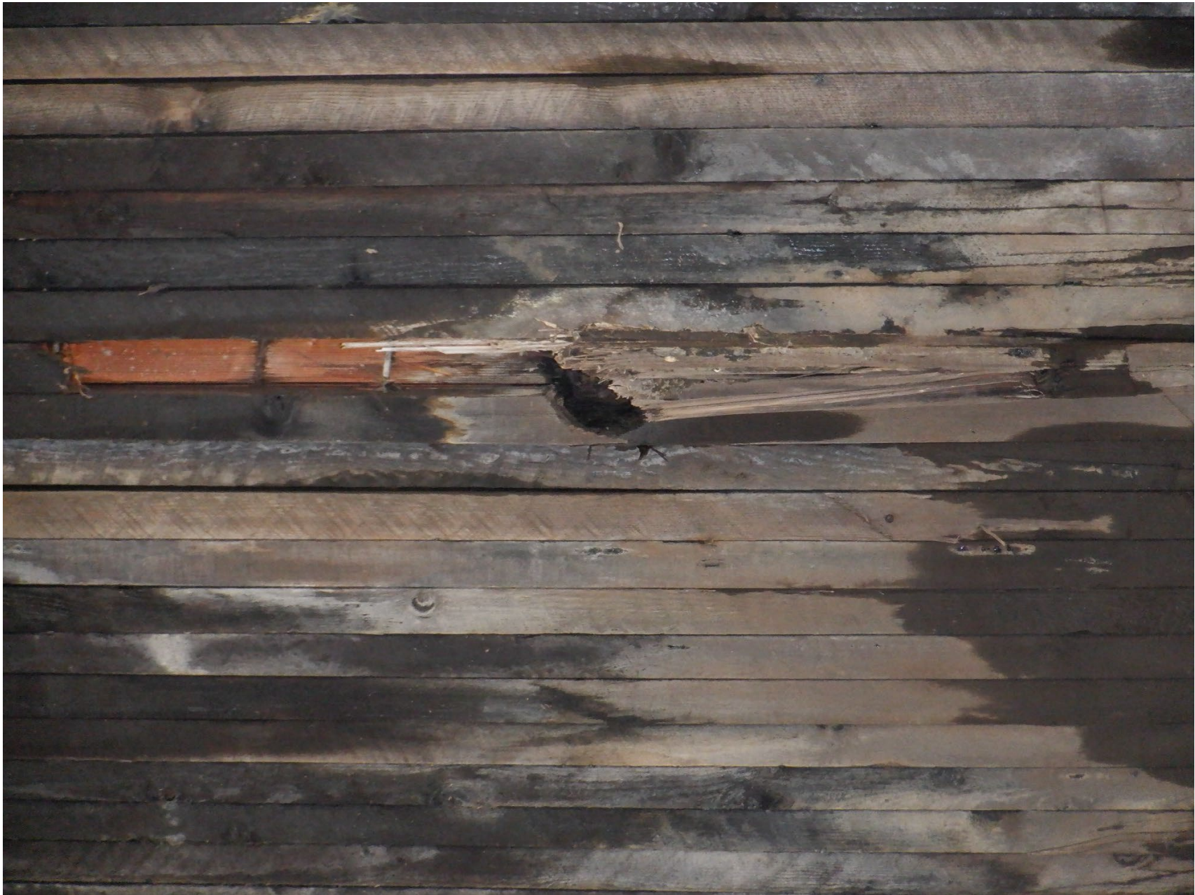
DECK BOARDS DAMAGED FROM SOIL BORING IN CENTER SPAN
