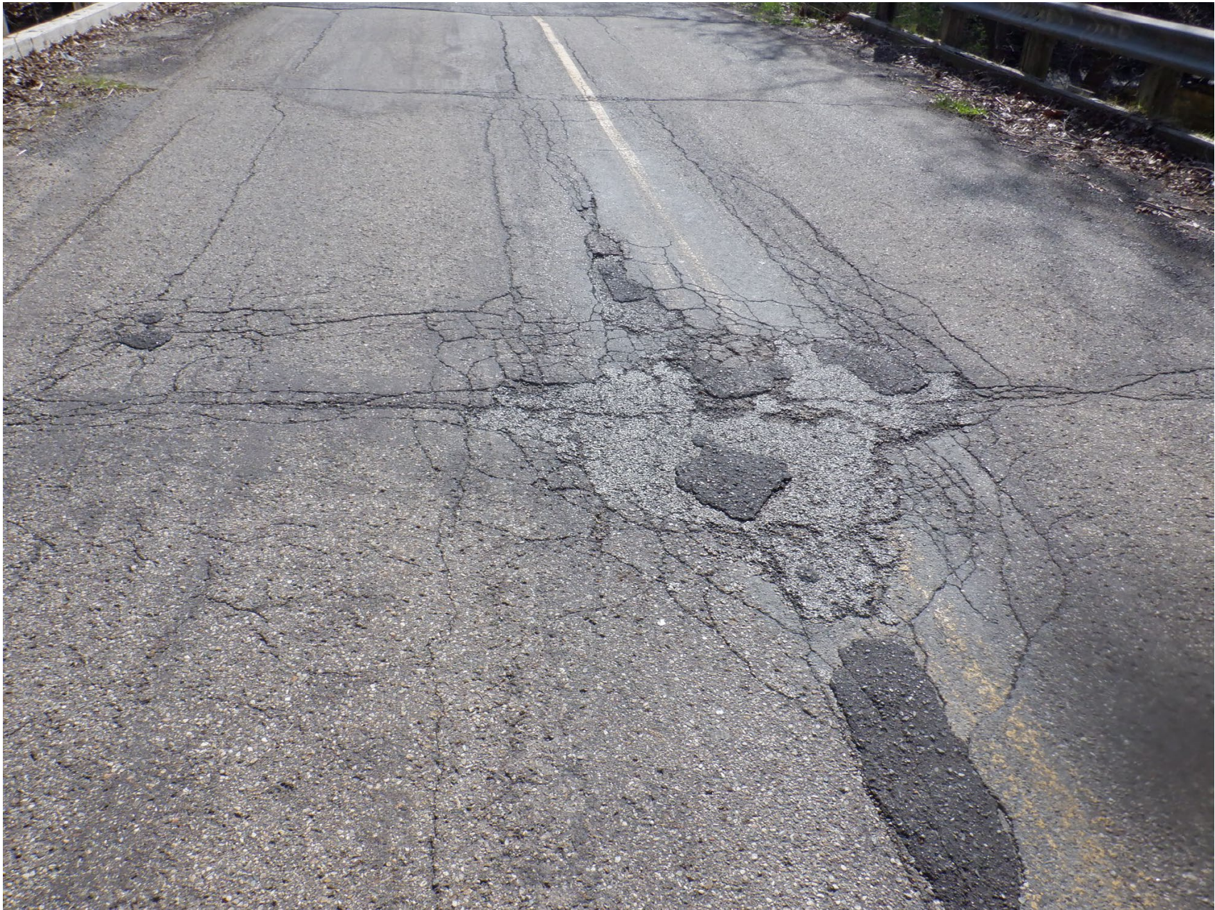
LONGITUDINAL AND ALLIGATOR CRACKS IN HMA SURFACE WITH SETTLEMENT AT CENTERLINE OVER WEST PIER
