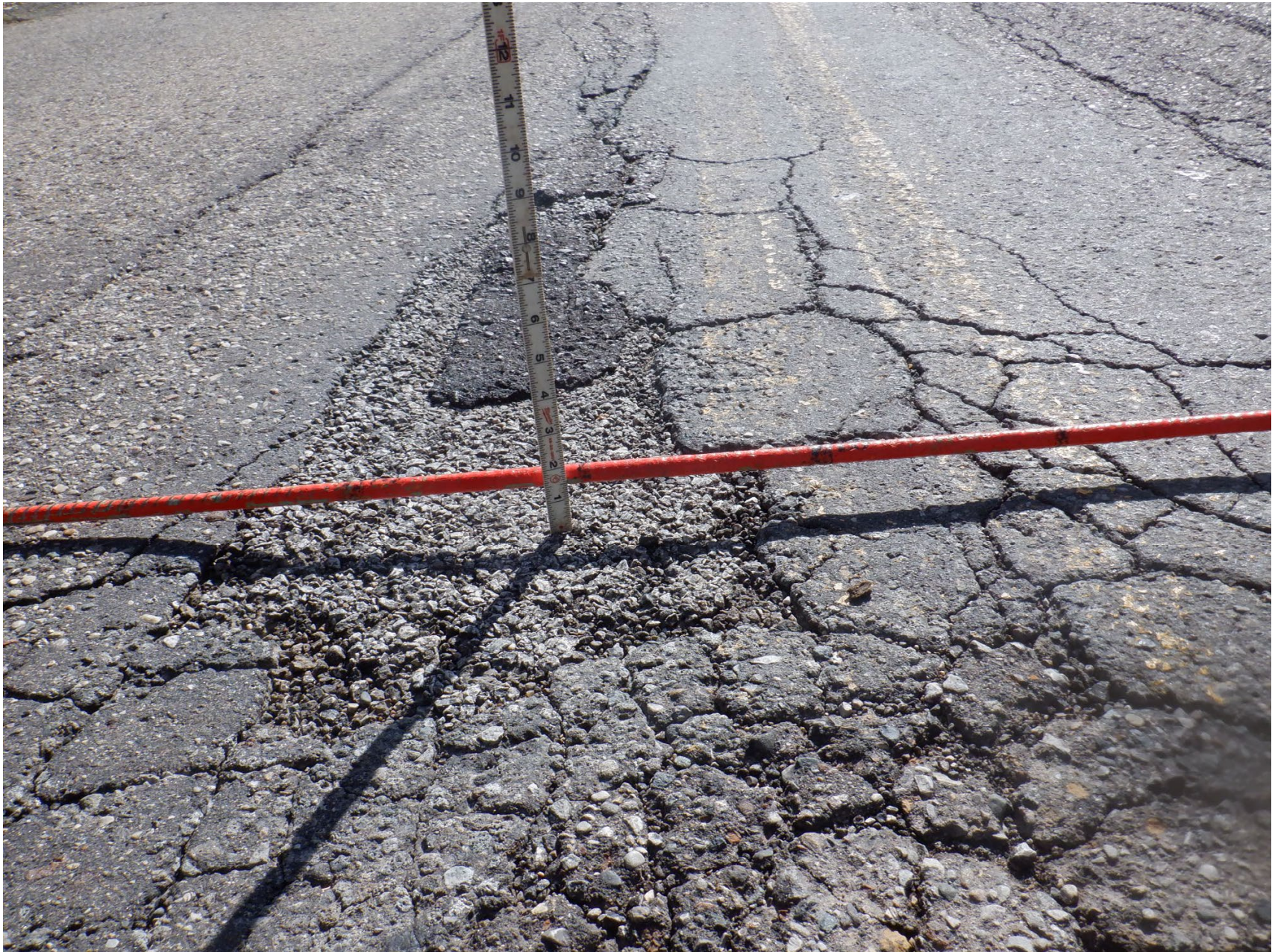
UP TO 1.25" SETTLEMENT AT CENTERLINE OVER WEST PIER
