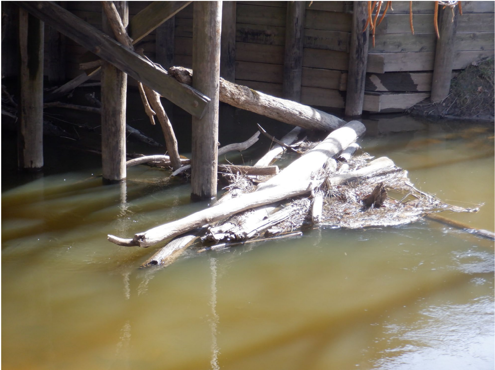
DEBRIS CAUGHT ON EAST PIER AND IN EAST SPAN
