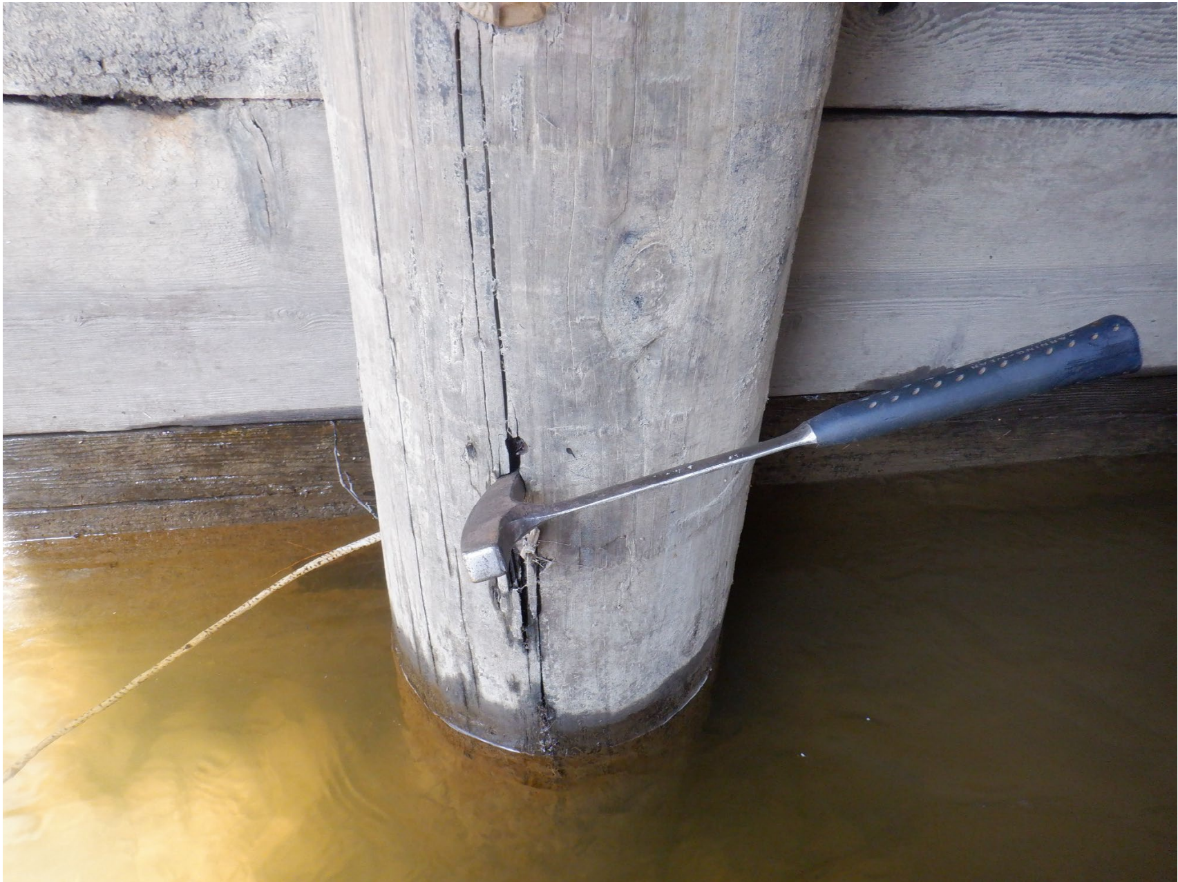
WEST ABUTMENT PILE 3S CHECKING WITH DECAY STARTING NEAR WATERLINE
