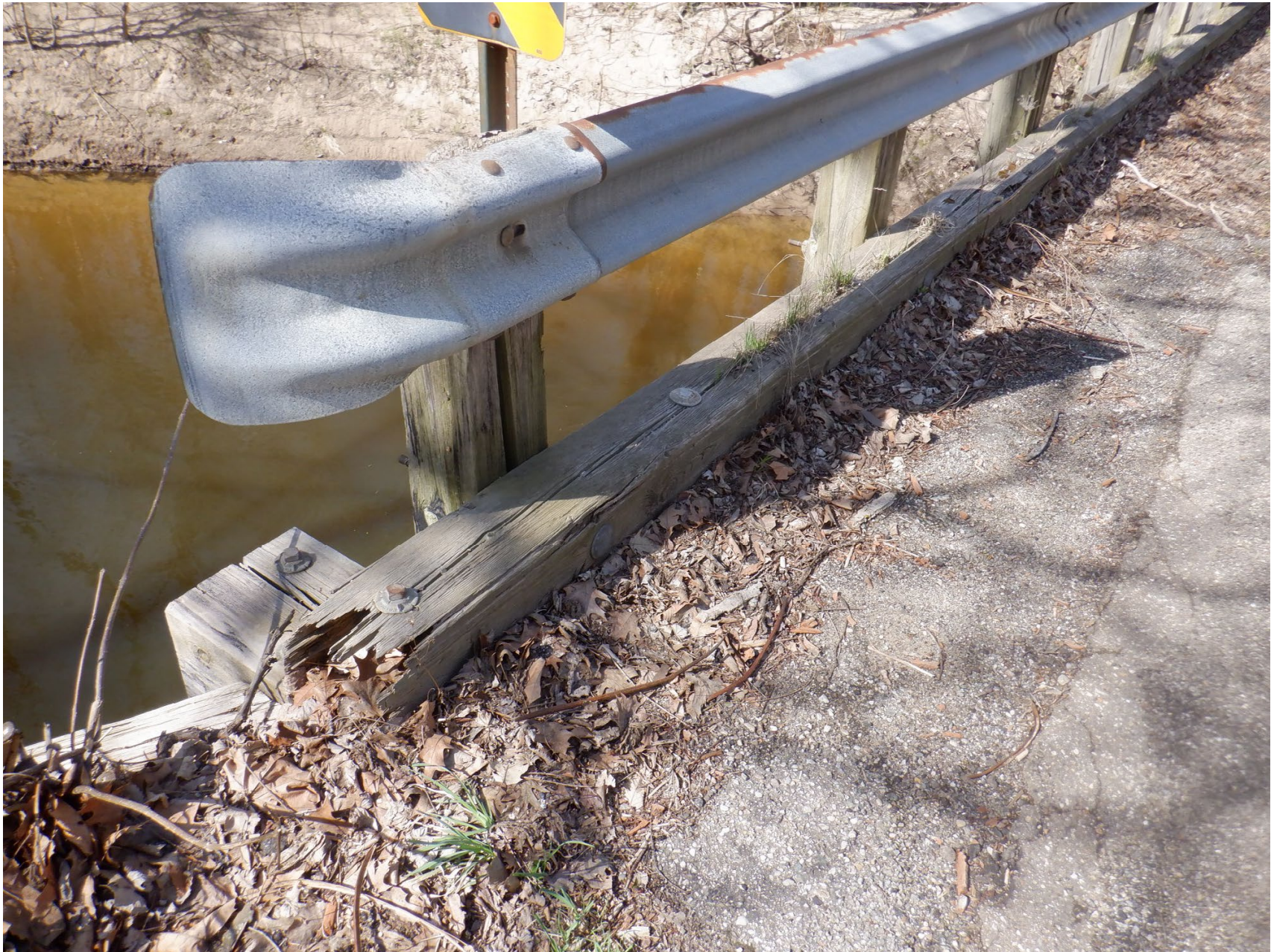
EAST END OF SOUTH BRUSH BLOCK ROTTING
