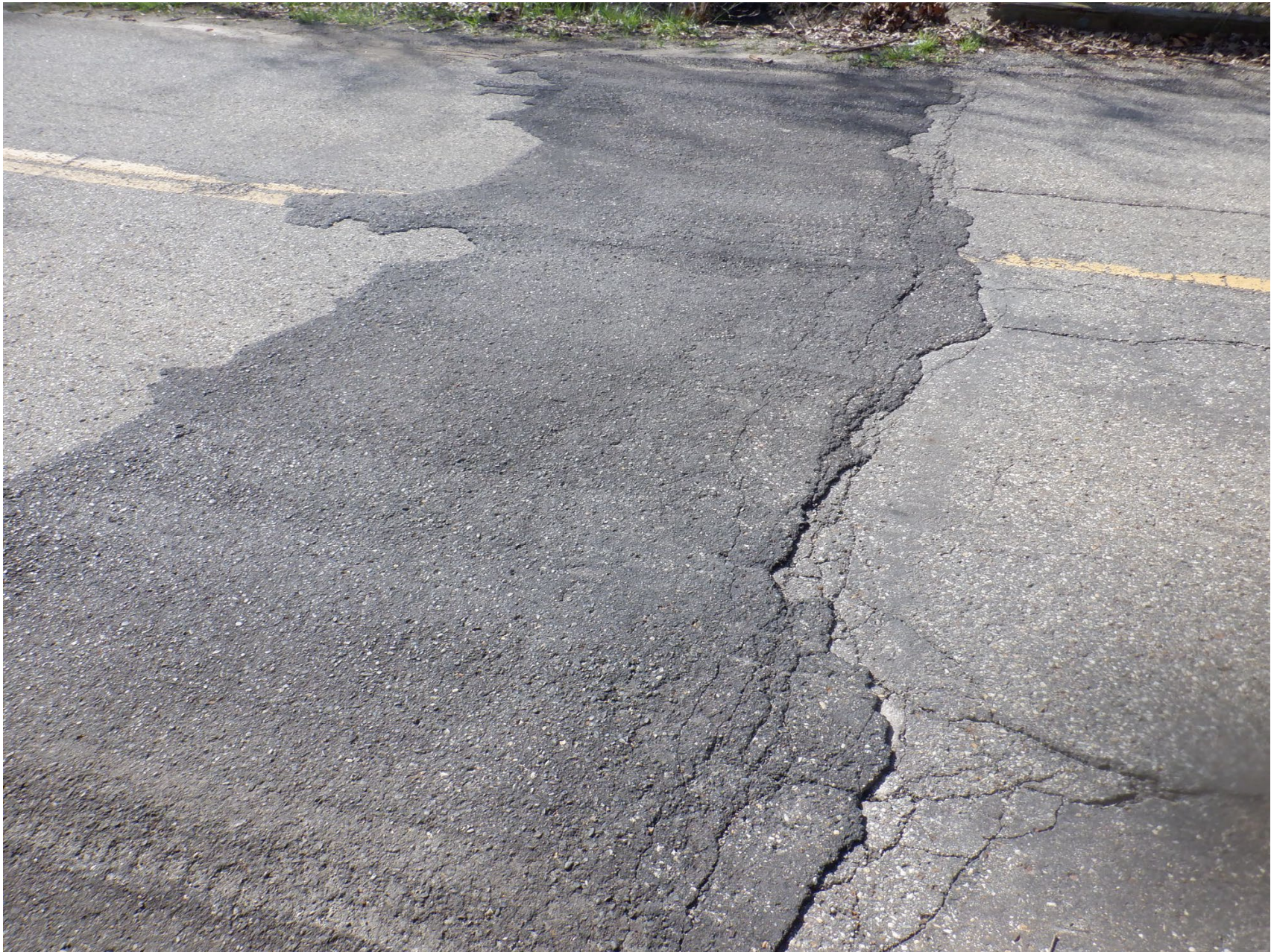
NEWER HMA WEDGING ON EAST APPROACH
