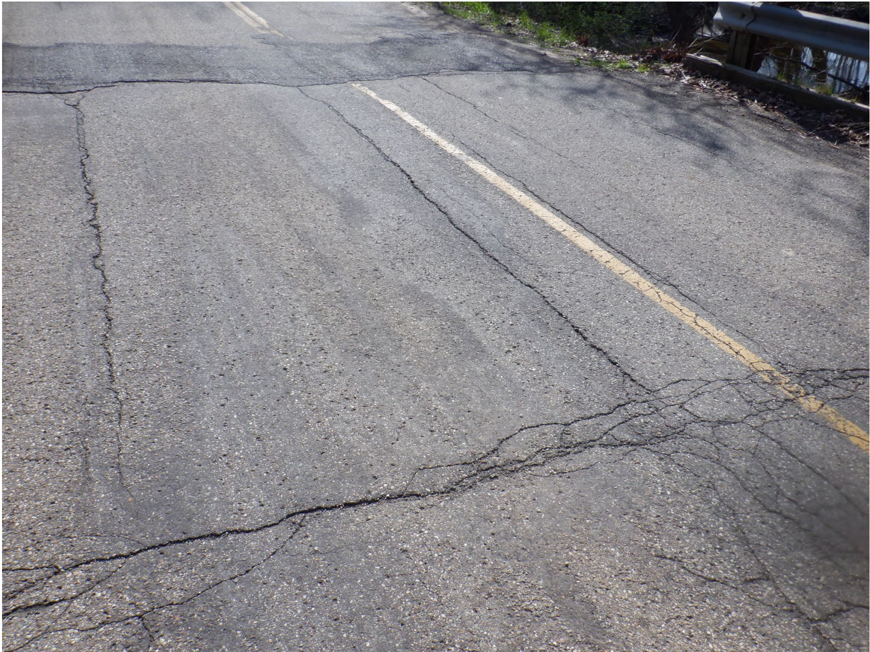
LONGITUDINAL CRACKS IN EAST SPAN, TRANSVERSE AND ALLIGATOR CRACKS OVER EAST PIER
