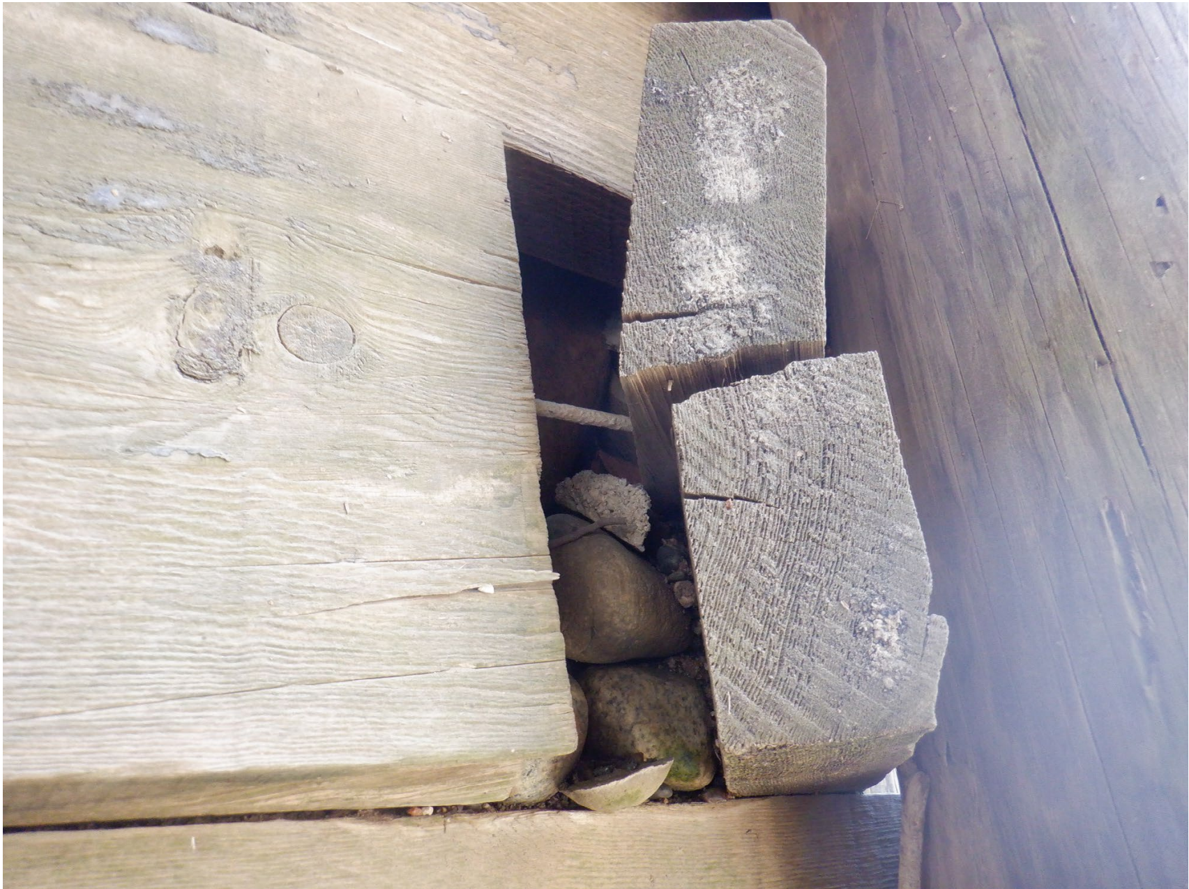
GAP IN BACKWALL BOARDS AT SOUTHEAST ABUTMENT CORNER
