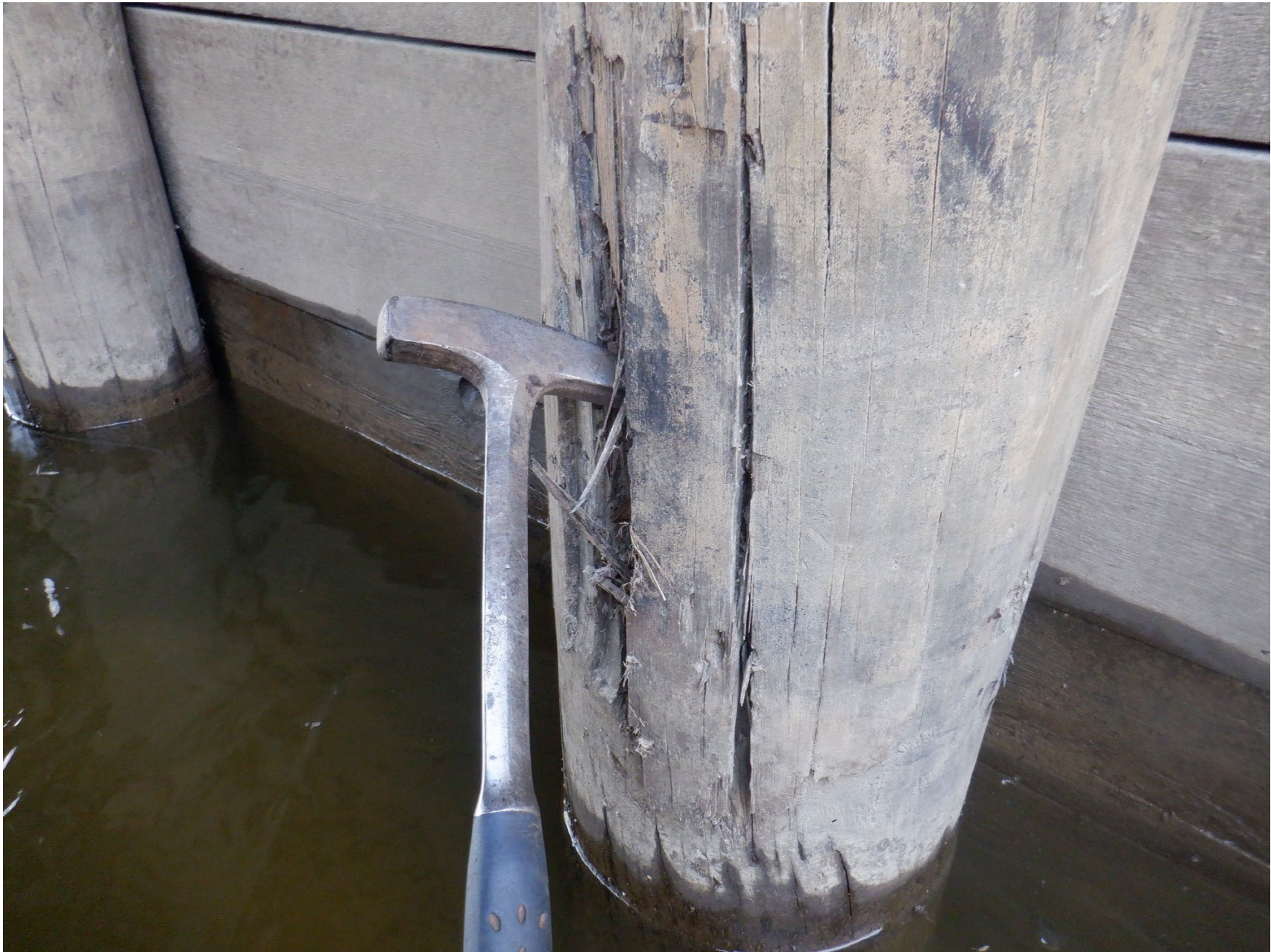
WEST ABUTMENT PILE 2N OUTER COVER CRACKED WITH ROT 2" DEEP ABOVE WATERLINE
