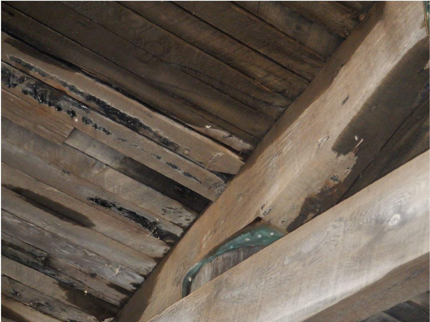
BROKEN DECK BOARDS ON WEST SIDE OF WEST PIER NEAR CENTERLINE
