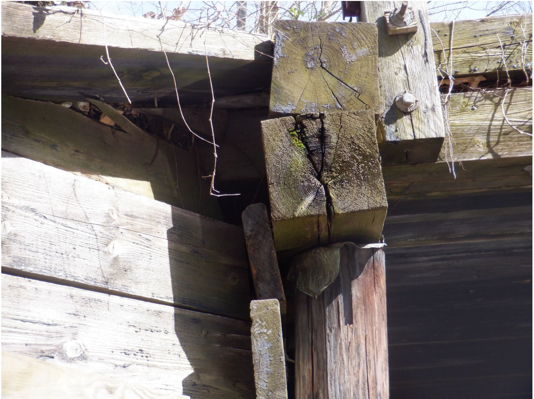
SPLIT AT SOUTH END OF WEST ABUTMENT CAP
