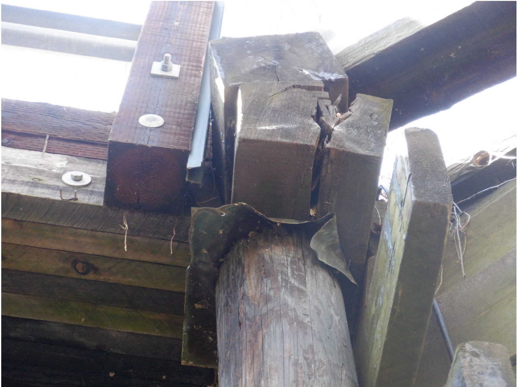
NORTH END OF WEST ABUTMENT CAP SPLIT AND ROTATED BACK
