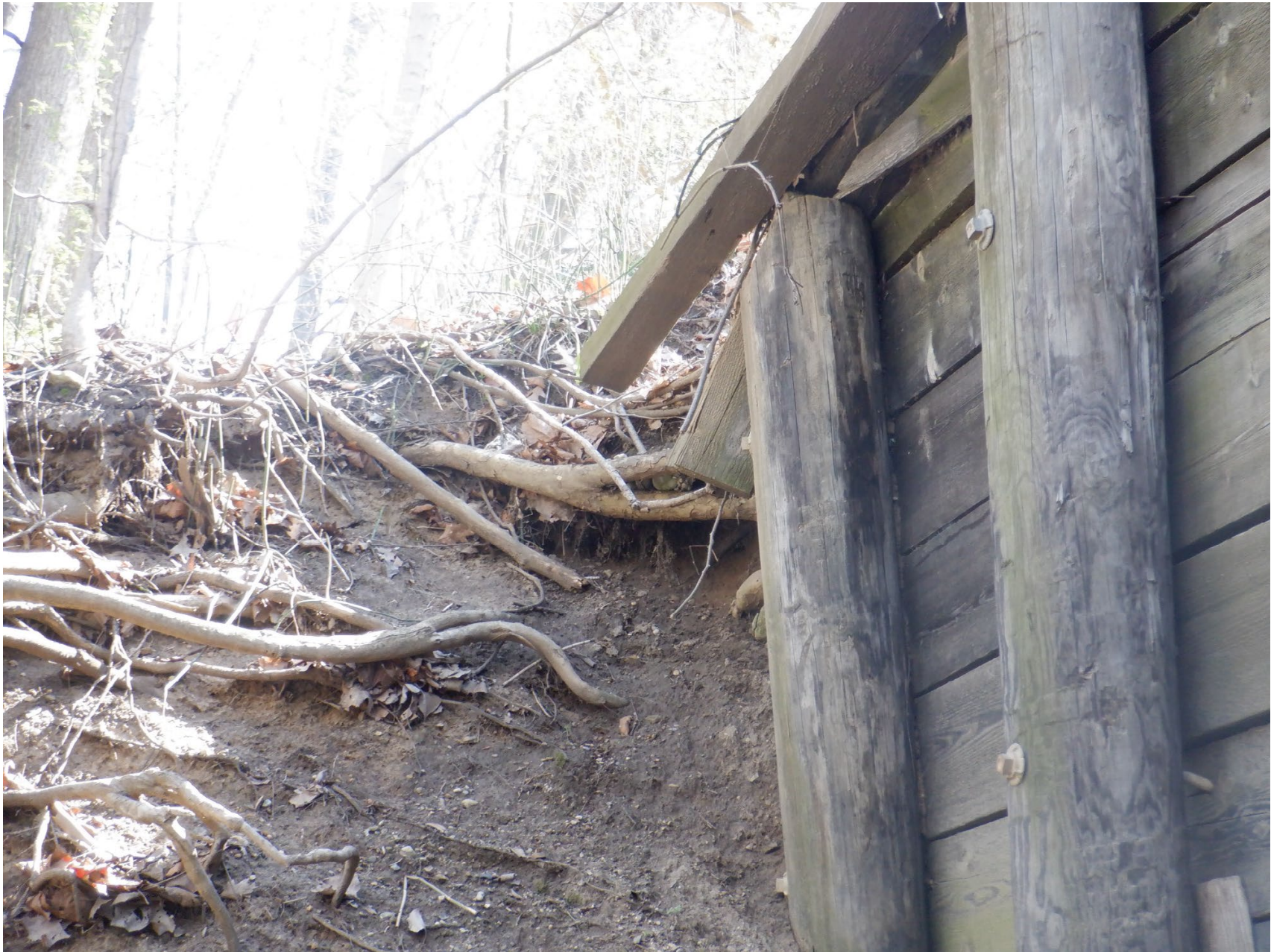
RAW SLOPE IN NORTHEAST QUAD, END OF WINGWALL CAP SPLIT
