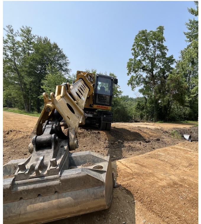
PIPE REPLACEMENT ON 64TH AVENUE IN PAW PAW
